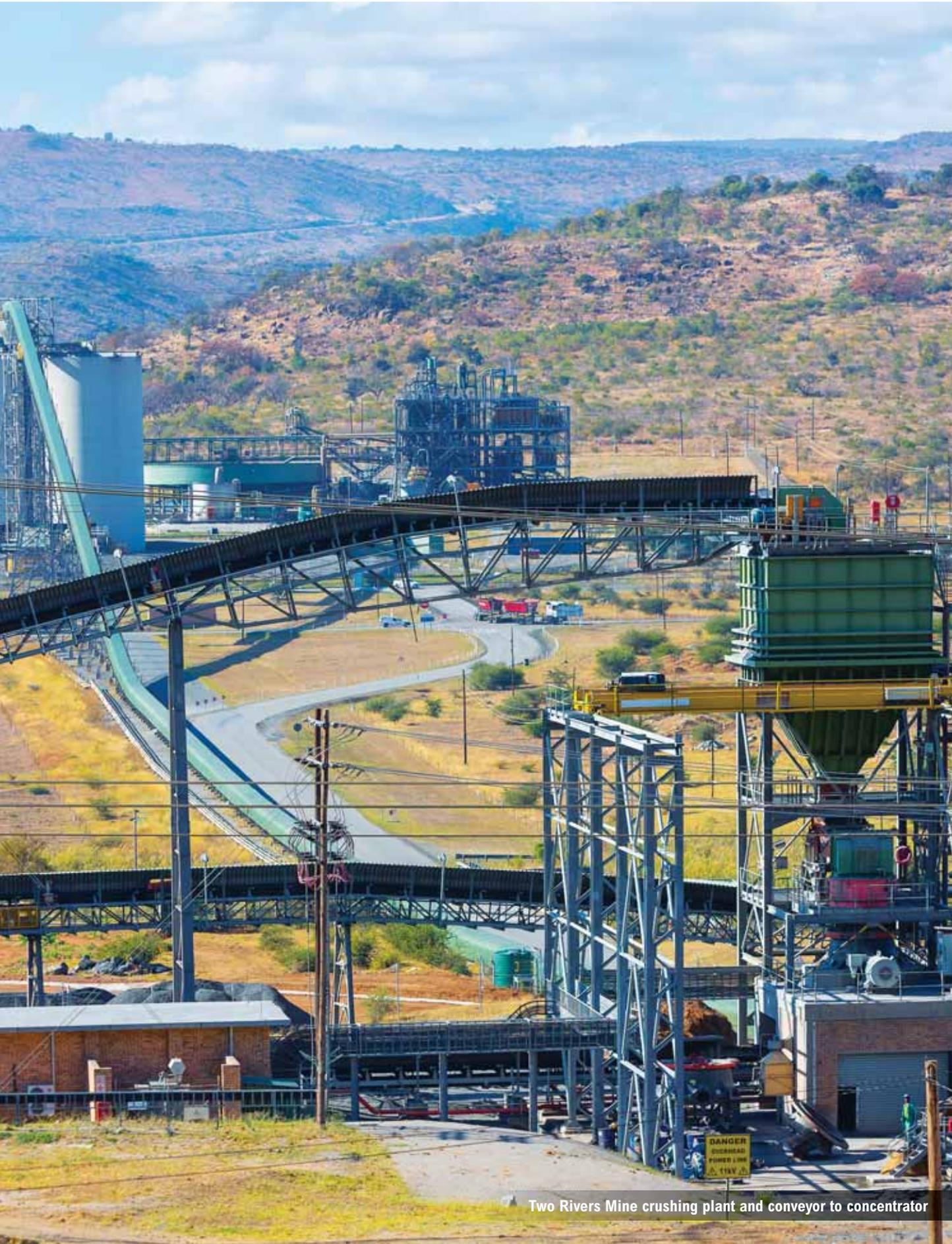
Two Rivers Mine crushing plant and conveyor to concentrator
