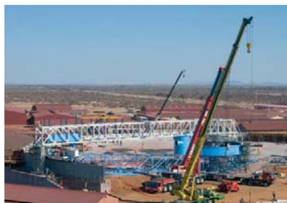
Construction of new thickener at Khumani
