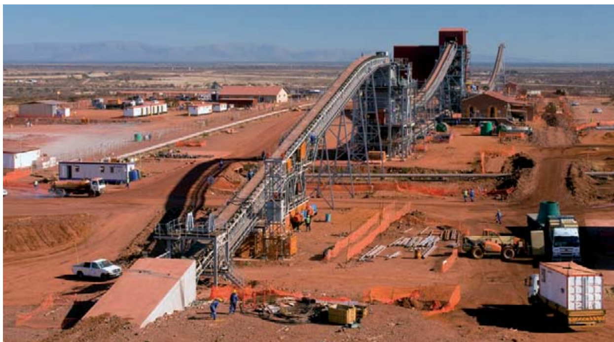
The King Primary and secondary crusher installation under construction at Khumani Mine
