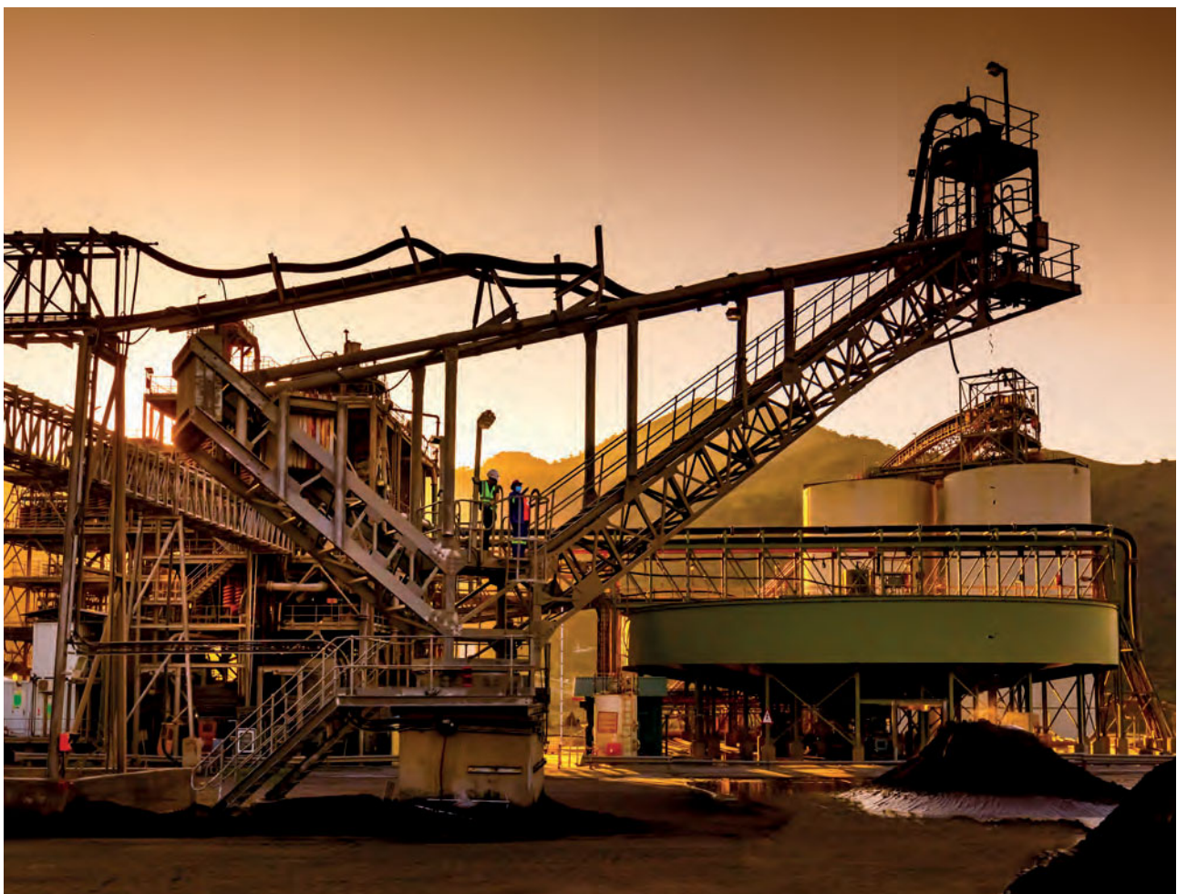
Two Rivers Platinum Mine.
