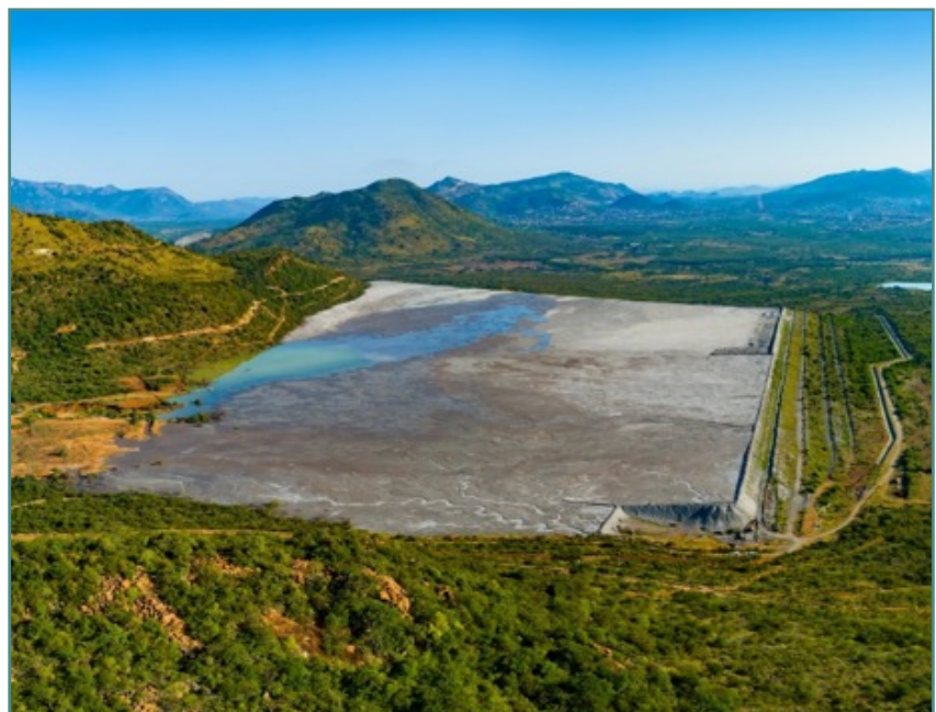
Figure 1-1: MPM tailings storage facility
