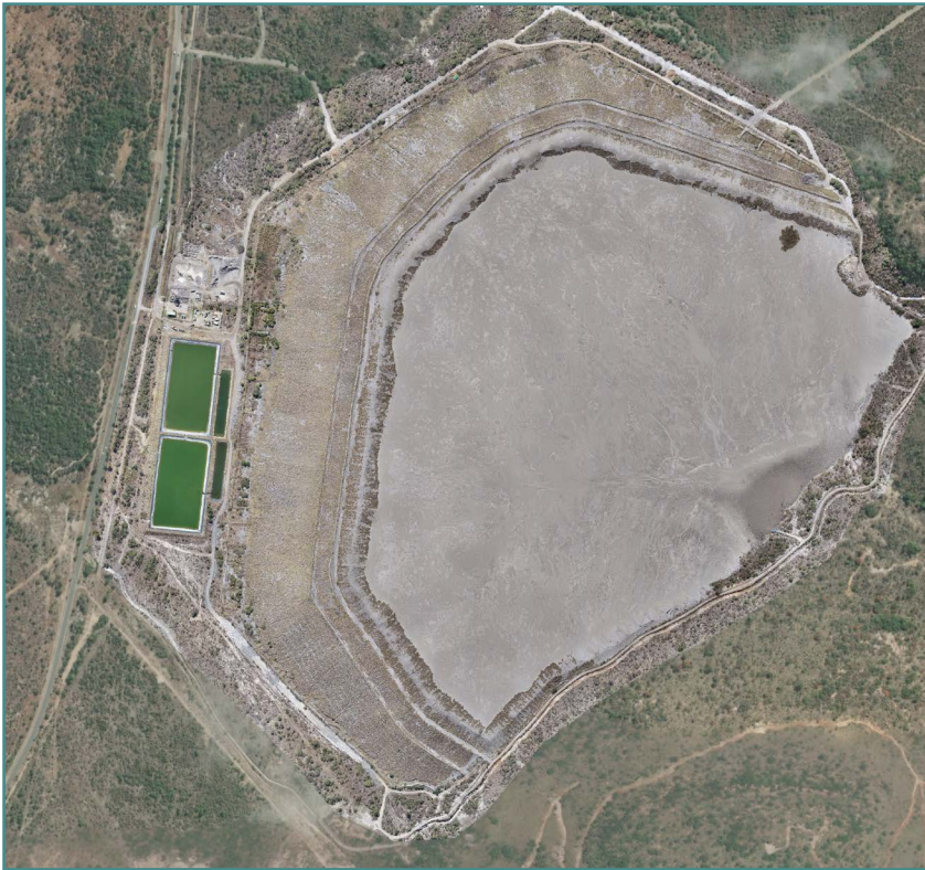
Figure 1-2: TRP tailings storage facilities locality map (Old TSF)
